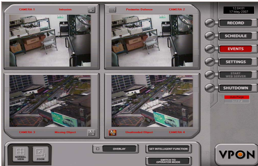
Fig. 2.1 Multiple camera view
